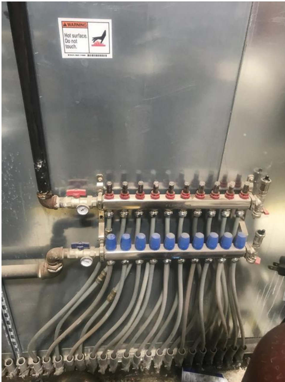
Hydronics Manifold
